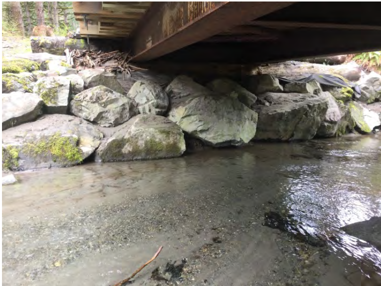
Left Bank Abutment when facing downstream
