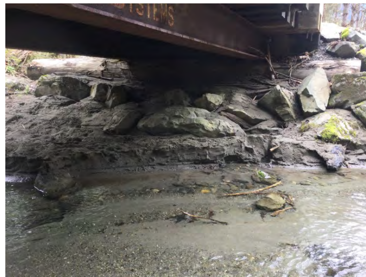
Right Bank Abutment when facing downstream
